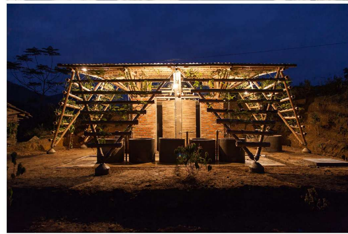
the toilet block brightly illuminated at night
